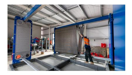
Over the past few weeks Melbourne-based Environmental Technology Solutions has been installing Parakiore's unique Waste Water Heat Recovery System in a separate plant room on St Asaph Street.
