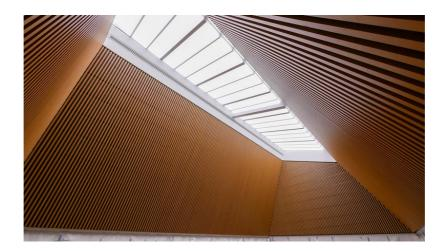
In the photos above you can see the lining going on the five large 13m x 7m skylights over the pools. These diffuse the incoming natural light, so it won't disturb the swimmers or tv cameras below during events. The use of natural light also reduces the number of lights that need to be switched on during the day.
