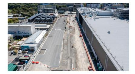
One of the most noticeable changes you will soon see is the asphalt being poured for the first car park on the western side of the building. Once this is completed earthworks will continue on the St Asaph St entrance to the facility.
