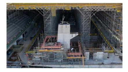
At the southern end of the aquatics building, formwork is being constructed and reinforcing steel is being tied on the dive tower, ahead of the concrete pours for the three and five metre dive platforms.
